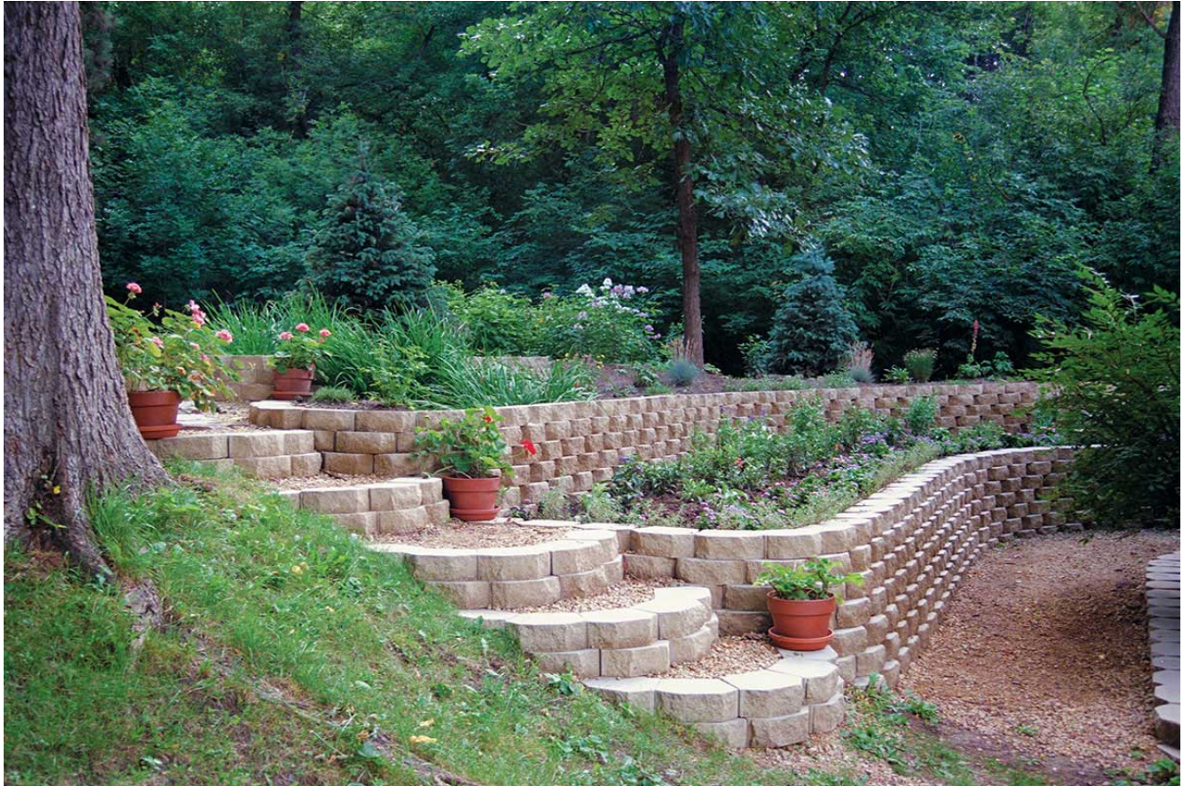
Example of terraced block retaining walls:
