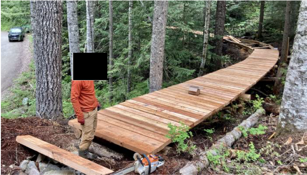
Bridging Work on Flashback. Built to the width required for the Adaptive Mountain Bike Blue Trail standard (June 2024)
