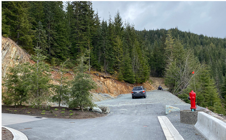
Figure 4. View south from driveway
