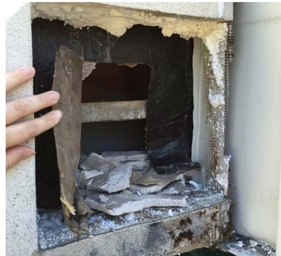
Photo A1-5 Pool - Exploratory Recess No.2
