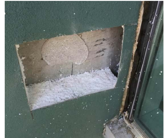
Photo A1-2 Pool - Exploratory Recess No.1
