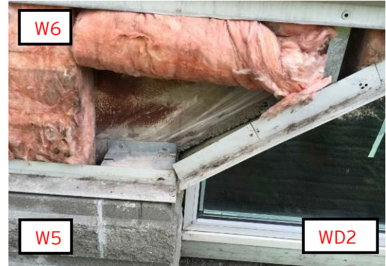
Photo A1-23 Ice Arena - East Elevation - Exploratory Recess No.11 - Exterior
