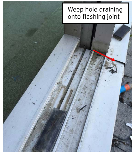
Photo A1-10 Pool Window - West Elevation Exploratory Recess No.5
