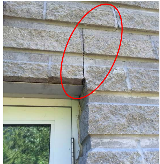
Photo A1-15 Fitness Centre - West Elevation
