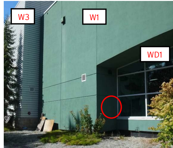
Photo A1-1 South Elevation Adjacent to Curtain Wall Windows
