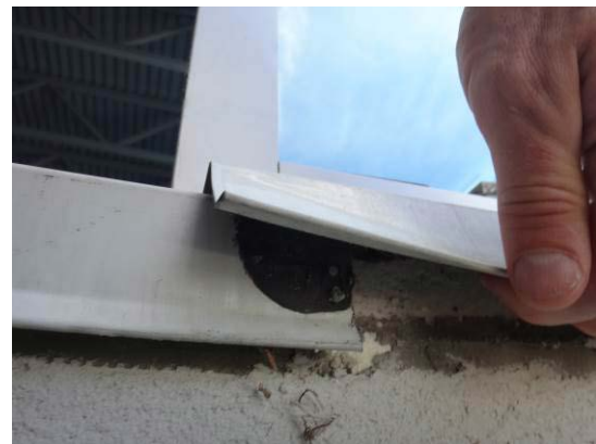
Photo A1-11 Pool Window - Exploratory Recess No.5
