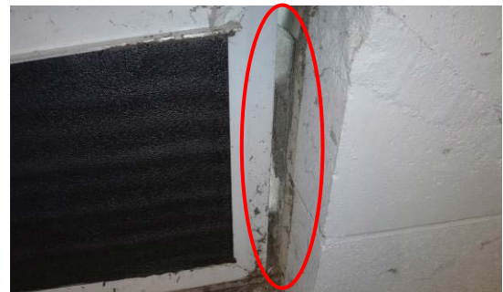
Photo A1-24 Ice Arena - East Elevation - Exploratory Recess No.11 - Interior
