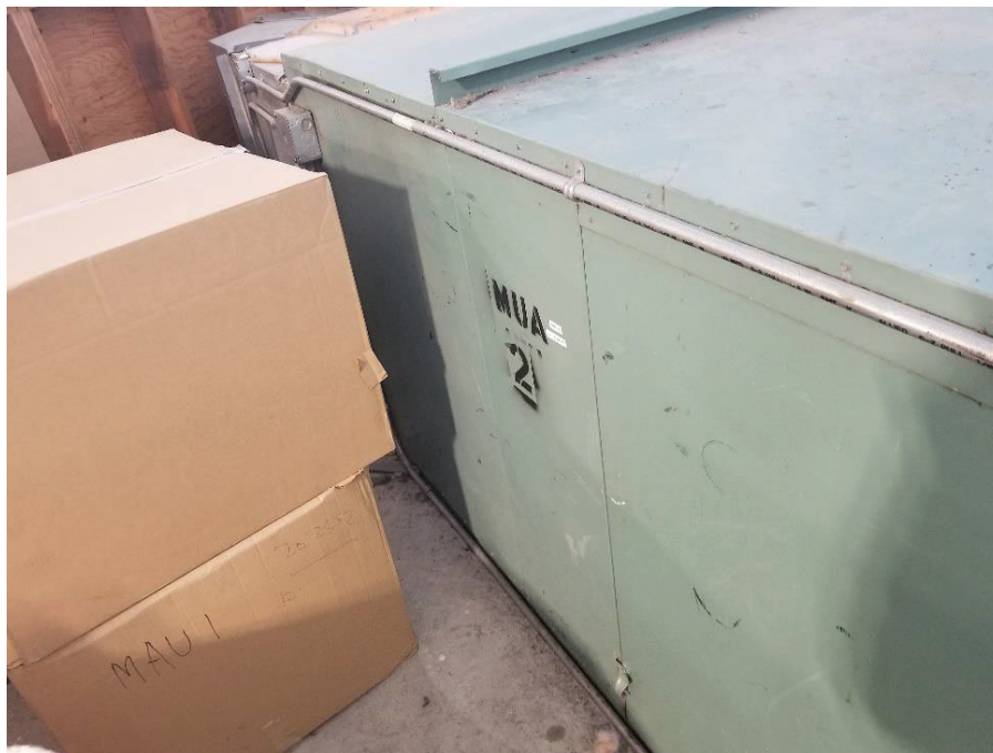
Figure 4: MUA-2 Site Photo
