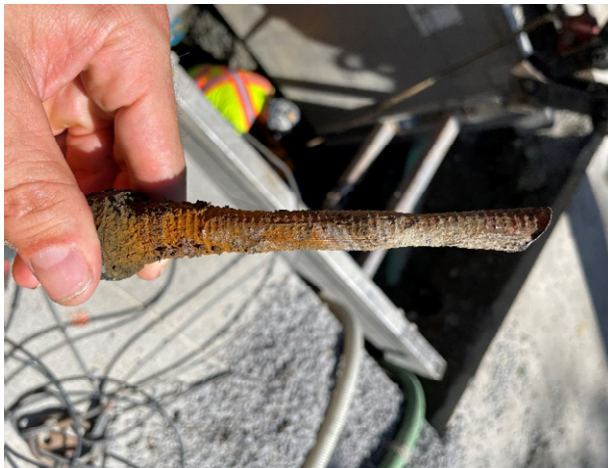
Photo 1 - Corroded Restraining Rod.
