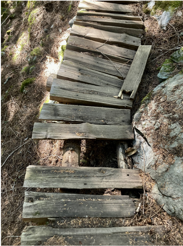
Example of decking repair on Get Over It trail, replaced by the WORCA crew. The WORCA Trail Crew splits their own decking - this is a great task for the team when the Fire Hazard is High/Extreme.
