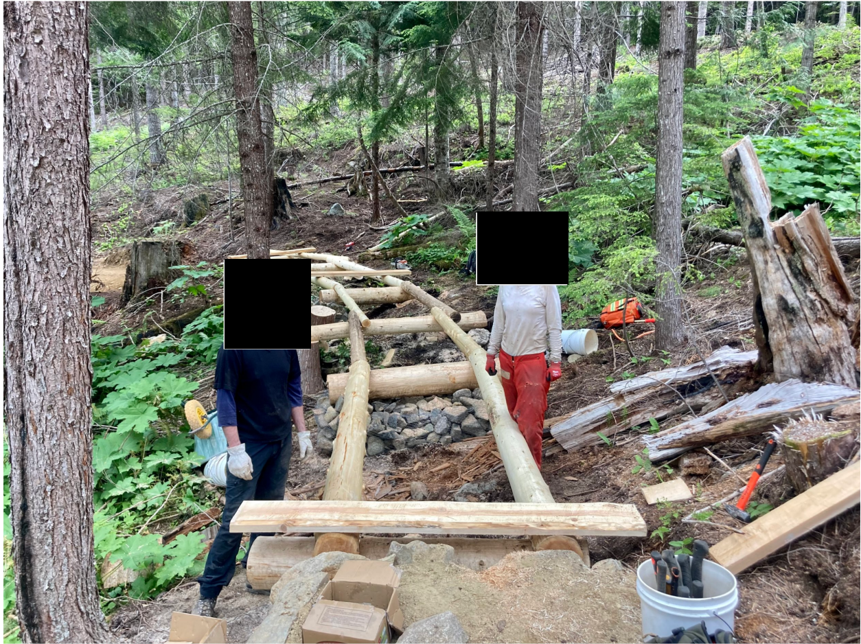
Installing/repairing new bridging
