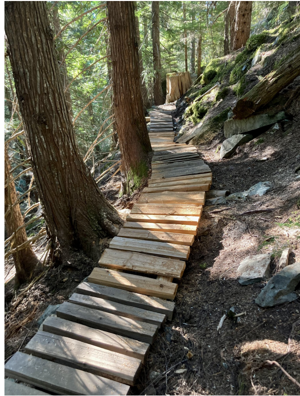
Example of decking repair on Get Over It trail, replaced by the WORCA crew. The WORCA Trail Crew splits their own decking - this is a great task for the team when the Fire Hazard is High/Extreme.
