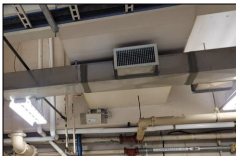
Figure 29: Distribution Ductwork
