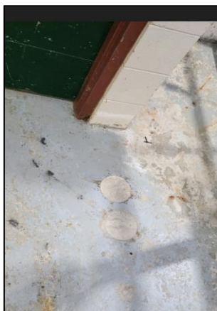
Figure 32: Sealed Pipework Penetrations from Decommissioned Heat Exchanger
