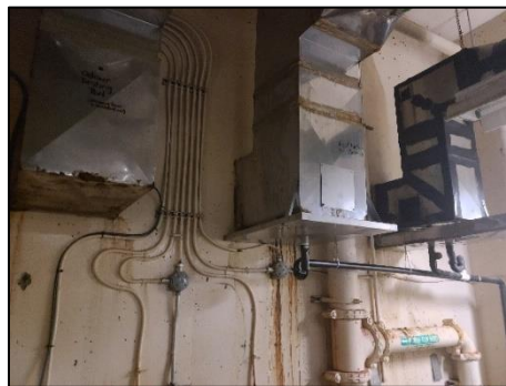
Figure 9: Supply and exhaust air
