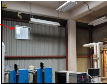
Figure 37: External Wall Opening
