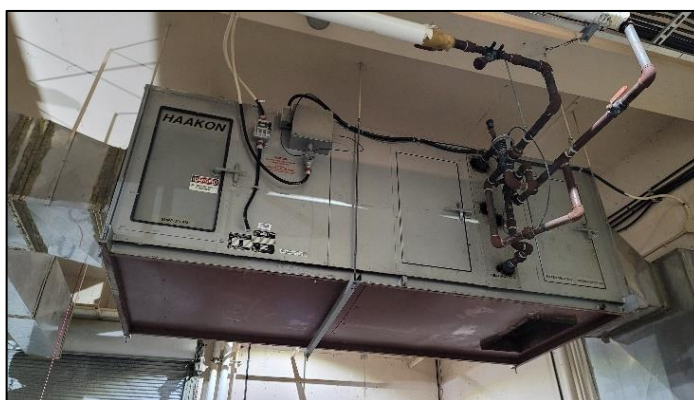
Figure 101: AHU-1
