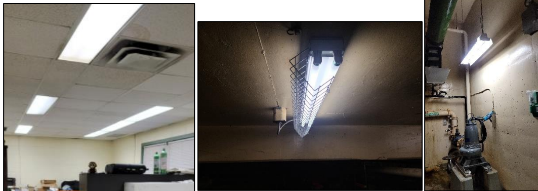
Figure 47: Typical T8-32W-2Lamp-4ft Recessed, Surface Mounted and Suspended Linear Fluorescent Luminaires
