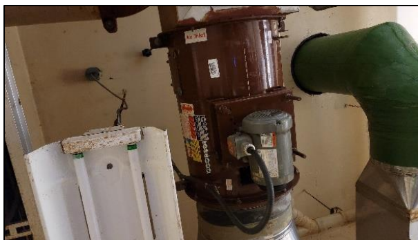
Figure 10: Exhaust Fan
