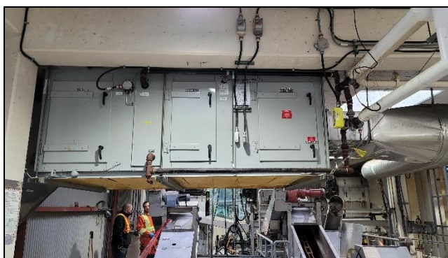
Figure 28: AHU-3 – HAAKON (100% Outdoor Air)
