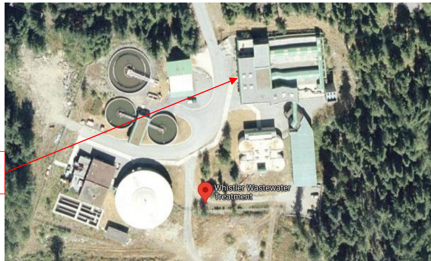
Figure 97: Aerial View of WWTP Rooftop, proposed location for PV installation
