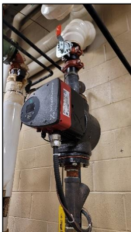
Figure 94: Existing MAGNA3 Pump
