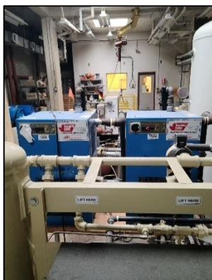
Figure 34: Air dryers
