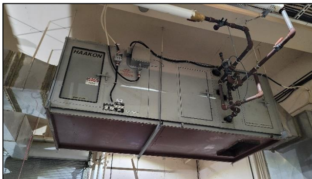
Figure 25: AHU-1 – HAAKON (100% Outdoor Air)
