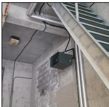
Figure 43: Unit Heater
