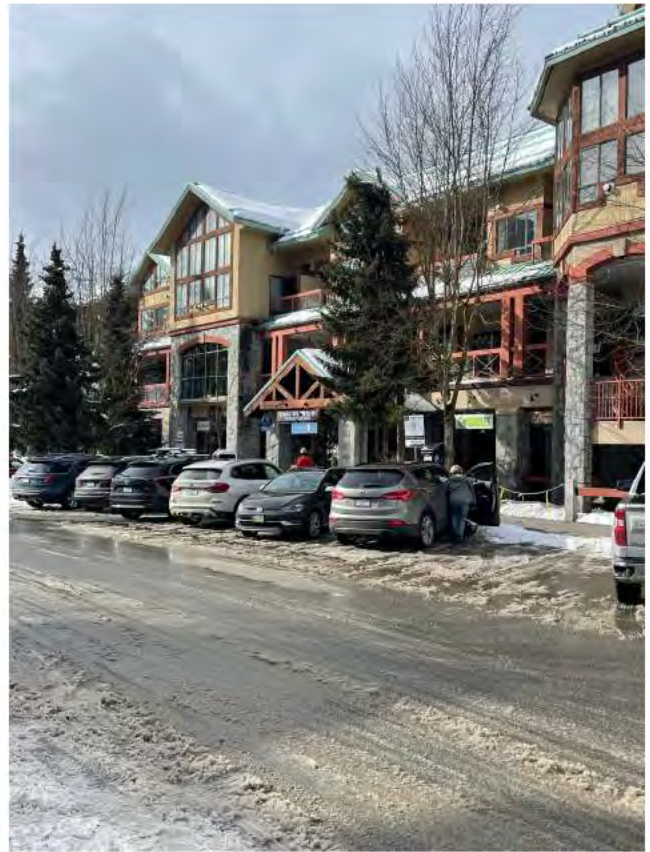
FRONT VIEW OF MARKET PAVILION
