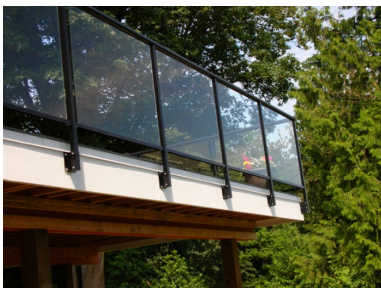
Balcony Guardrail example
