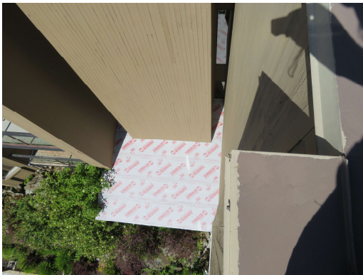
Photo 3 - Roof over elevator room with temporary self-adhesive membrane
