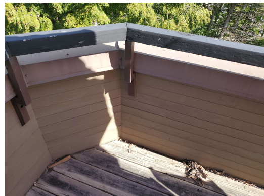
Photo 4 - Upper floor balcony decking.
