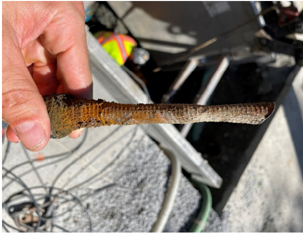
Photo 1 - Corroded Restraining Rod.
