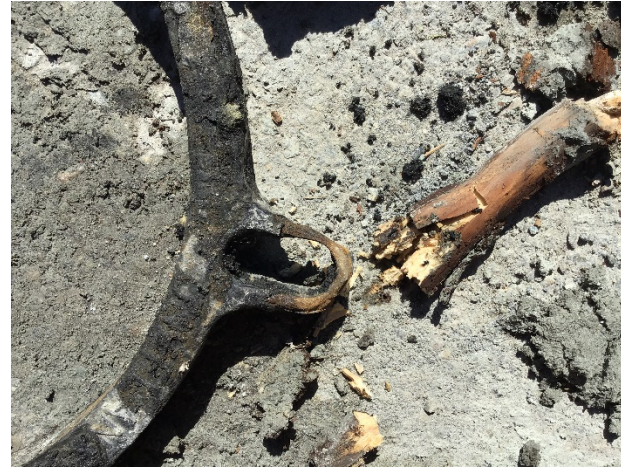
Photo 2 - Corroded Restraining Ring Ear.
