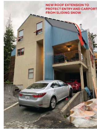
Figure 3 Diagram of proposed roof extensions impact on sliding snow and mitigation of risk.
