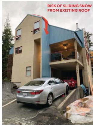
Figure 2 Photo of existing building illustrating exposure to sliding snow.
