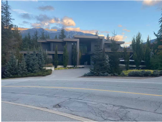
1. 7127 Nancy Greene Drive Contemporary Design; flat roof with roof elements coming to the ground; metal fascia with wood soffit.
