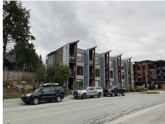
8. Cheakamus Multi Family 2 Standing seam angled roof, wood soffit, standing seam wall, together with post and beam.
