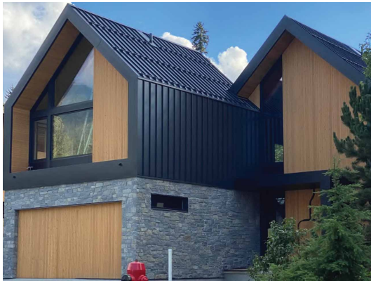
4. White Gold Property Gabled, standing seam metal roof extending down the wall.
