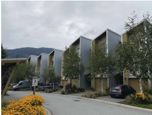
7. Cheakamus Multi Family 1 Standing seam angled roof, wood soffit, standing seam wall.
