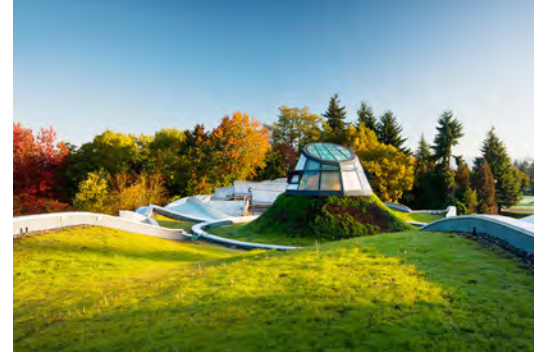
3 skylights integrated into the landscaped knoll providing daylight into the strata amenity
