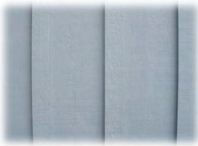
Existing Board and Batten siding
