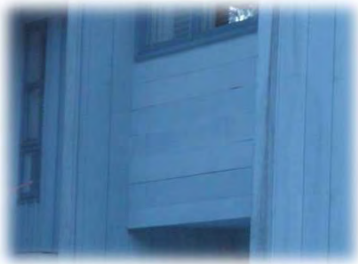
Existing 1X6 T+G Siding (vertical and horizontal)
