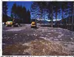
PHOTO - Lots 1 & 2 Looking West. Structural Fill Placed and compacted
