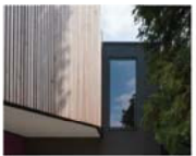
3 VERTICAL TIMBER SIDING (1" x 6" CEDAR)
