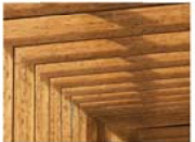
5 REPEATING GLULAM FRAME AT CANOPY
