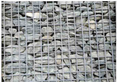
Entry Wall/ Gate - Gabion Wall Imagery
