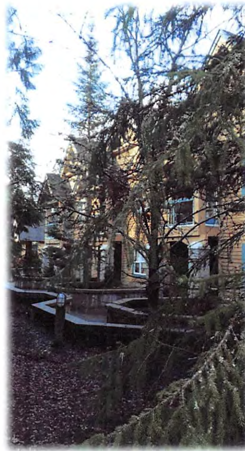
BUILDING 1 FROM NORTH END OF COURTYARD
