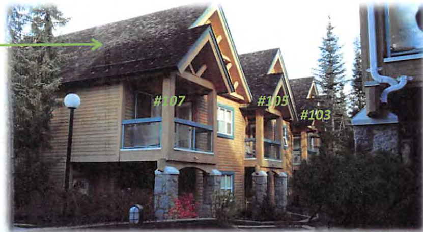
VIEW FROM WITHIN SITE SHOWING SOUTH END UNIT #107
