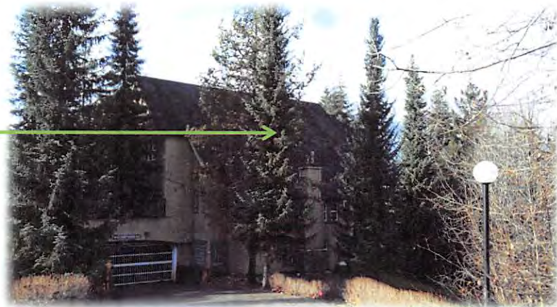
VIEW FROM DRIVEWAY North end of building #1
