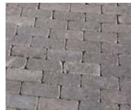
PAVING: precast concrete
