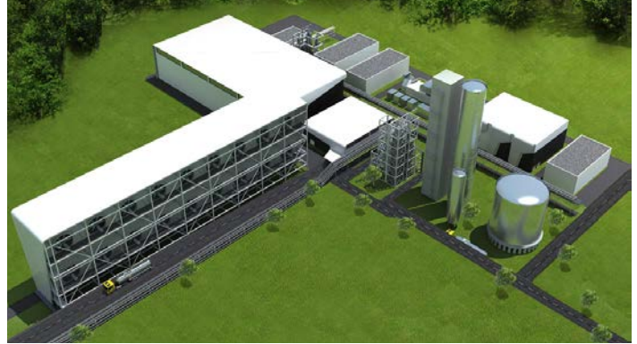
Graphical representation of a facility that would use Carbon Engineering's AIR TO FUELS™ process to manufacture roughly 2000 barrels per day of clean burning synthetic fuel.
