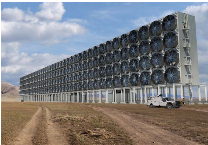
Rendering of Carbon Engineering's air contactor design. This unit would be one of several that would collectively capture 1M tonnes of CO 2 per year.
