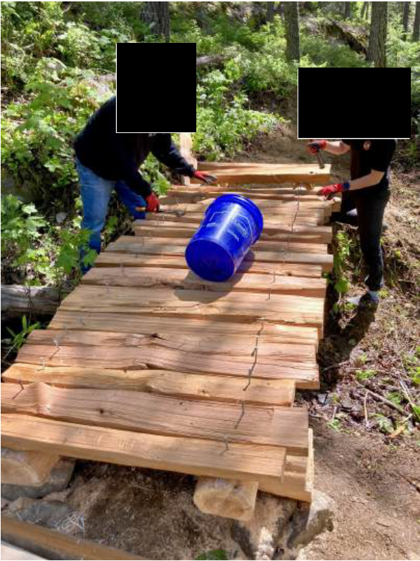
Whistler Adventure School (WAS) Sustainable Trail Building Class - Bridge Building (June 2024)
