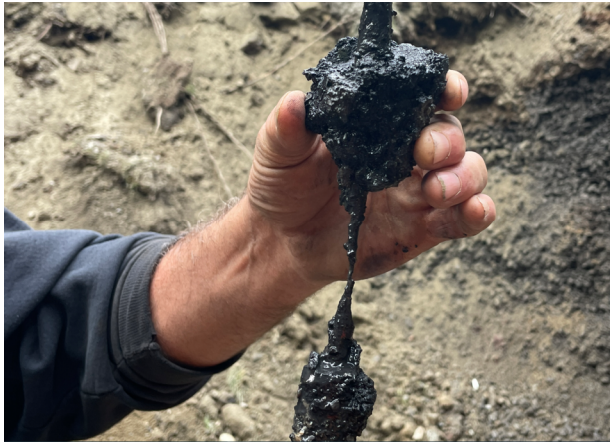
Photo 1 - Corroded Restraining Rod.
