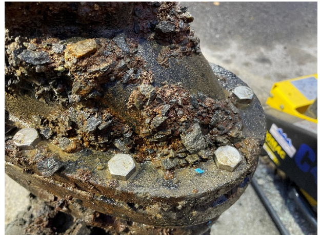
Photo 4 – W1-D Valve Bonnet Bolts
