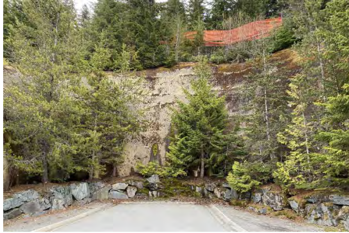
① SHOTCRETE WALL
